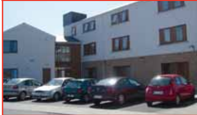
New Supported Living apartments in Sarsfield Park, Limerick
